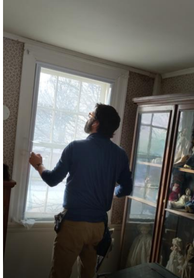
UV-blocking Film Installed on Windows.
